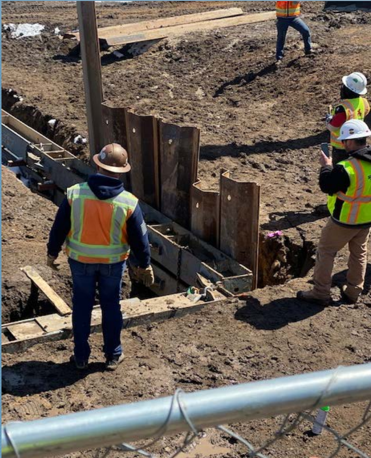
25' piling/shoring for Excavation Excavation dimensions = 40' x 60' x 23' depth
