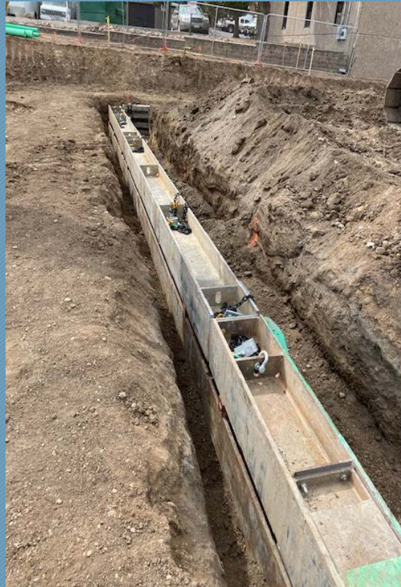
Hydraulic Support for Piling
