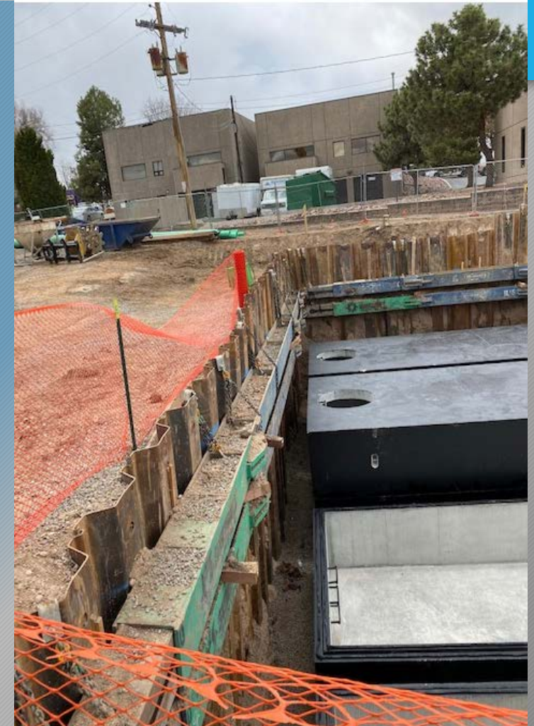
Overflow Tank Installation
