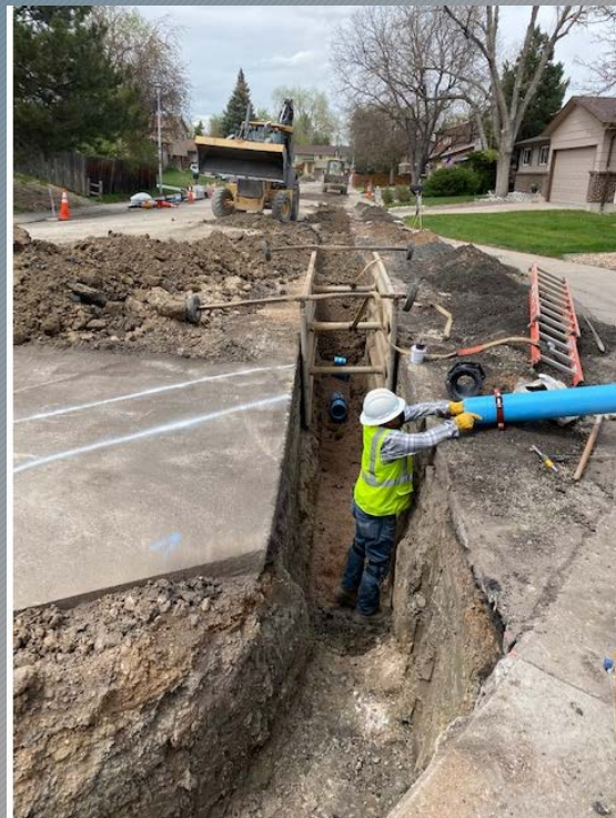
Flower Way 6" Water Trench
