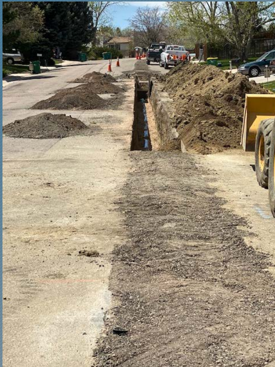
Walden Ave 12" Water Trench
