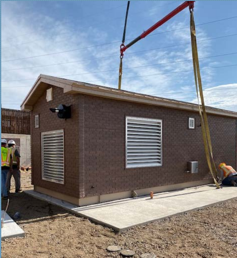
Setting Lift Station on Foundation
