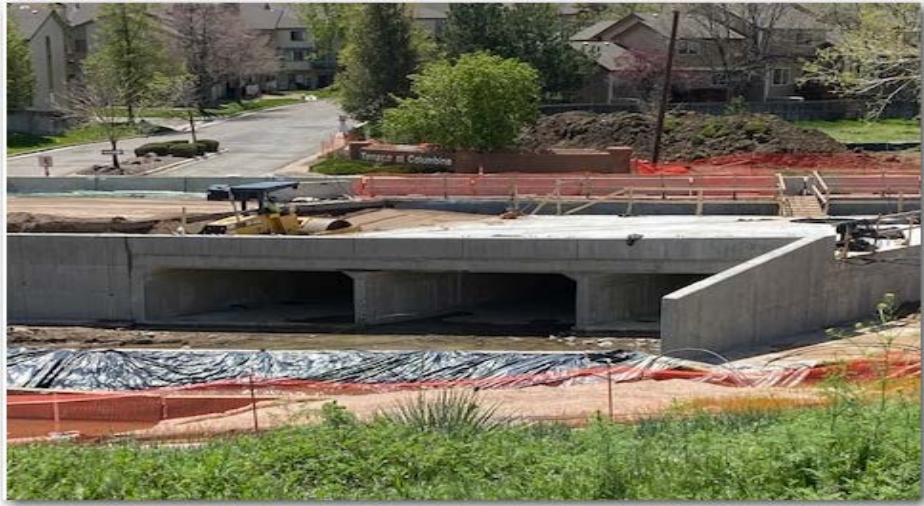
West Bound Coal Mine Near Completion
