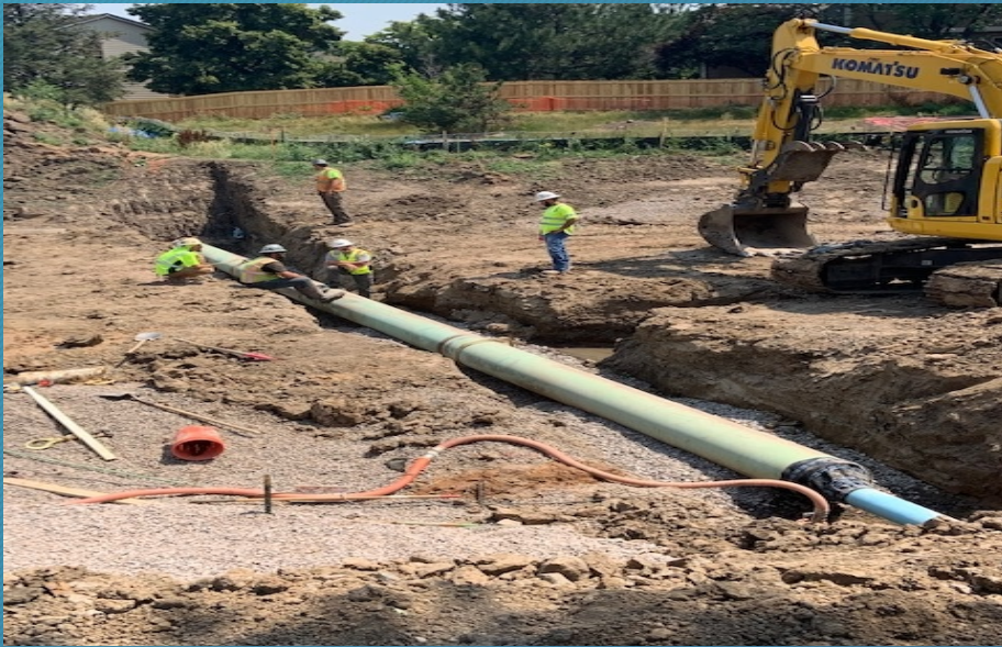
8" Sewer Main and Casing in Trench
