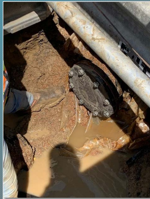
Removed tapping valve and installed plug on tapping sleeve
