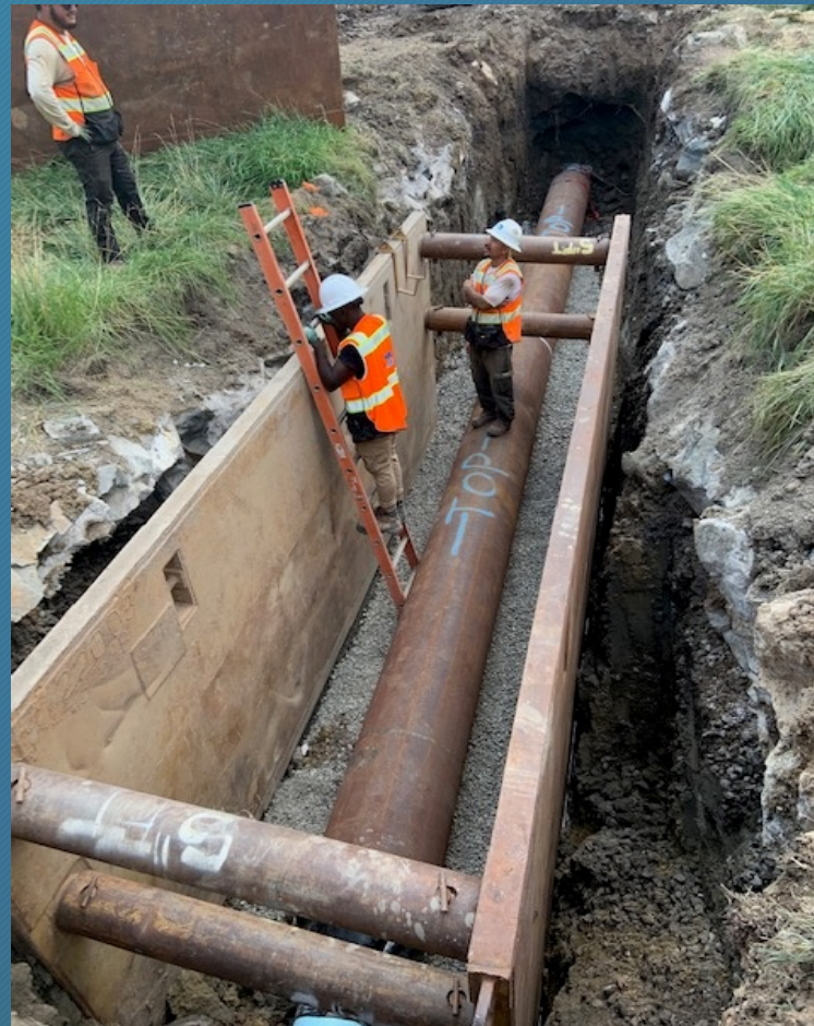
Steel casing in trench
