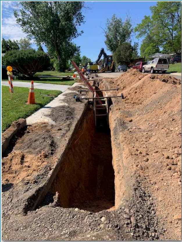
Construction in Depew
