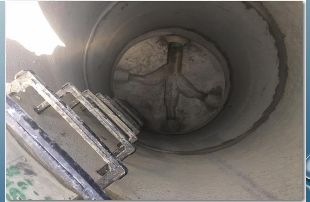
3-Way Service Connection to End Manhole
