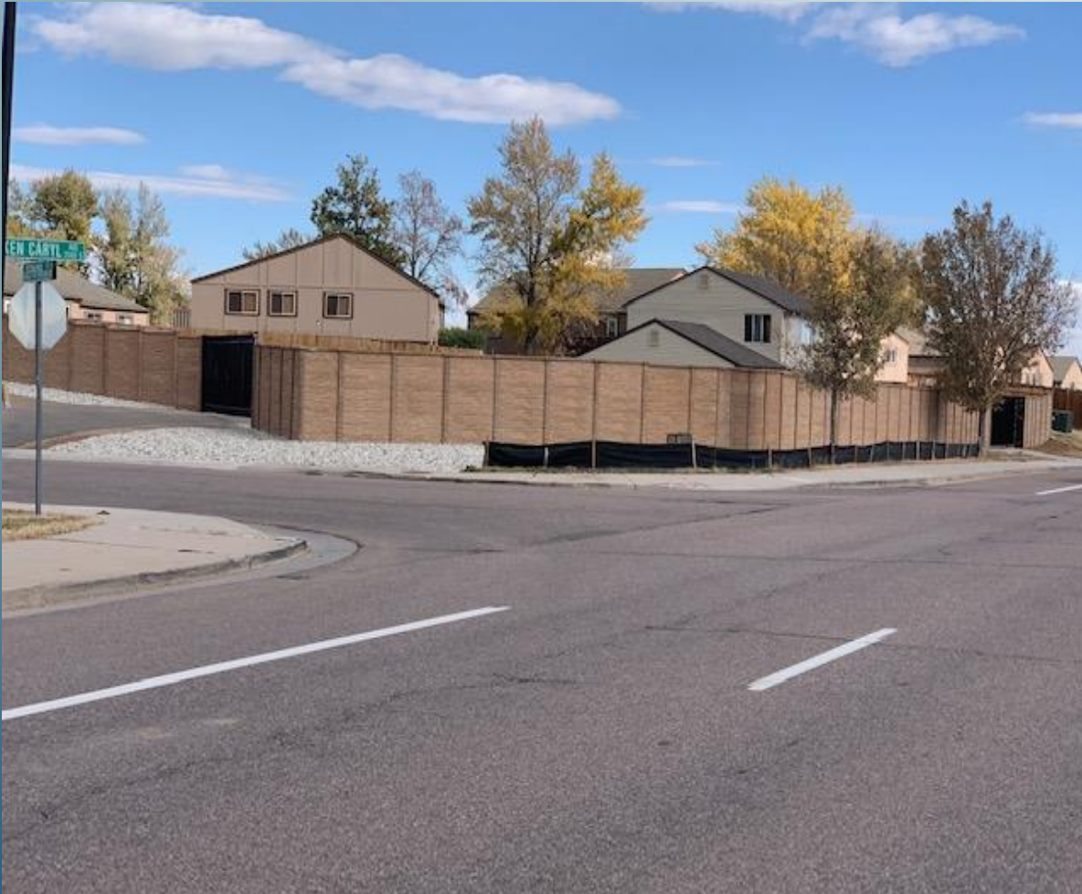
Completed fence and gates
