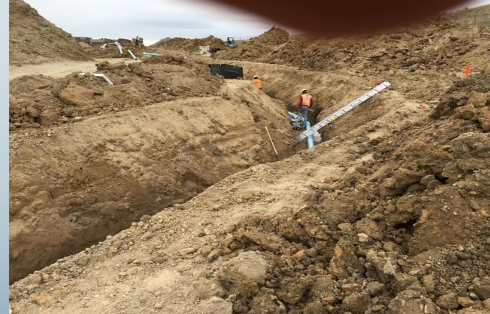
Water Main Trench
