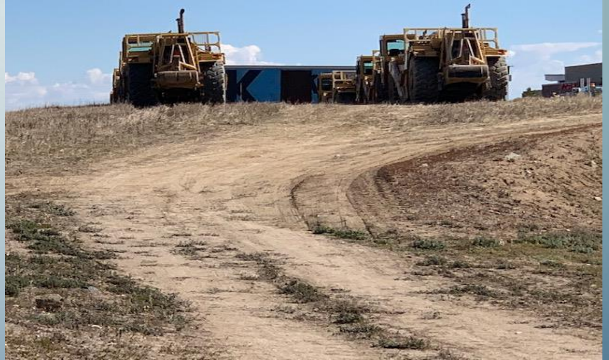
Earth Moving Equipment
