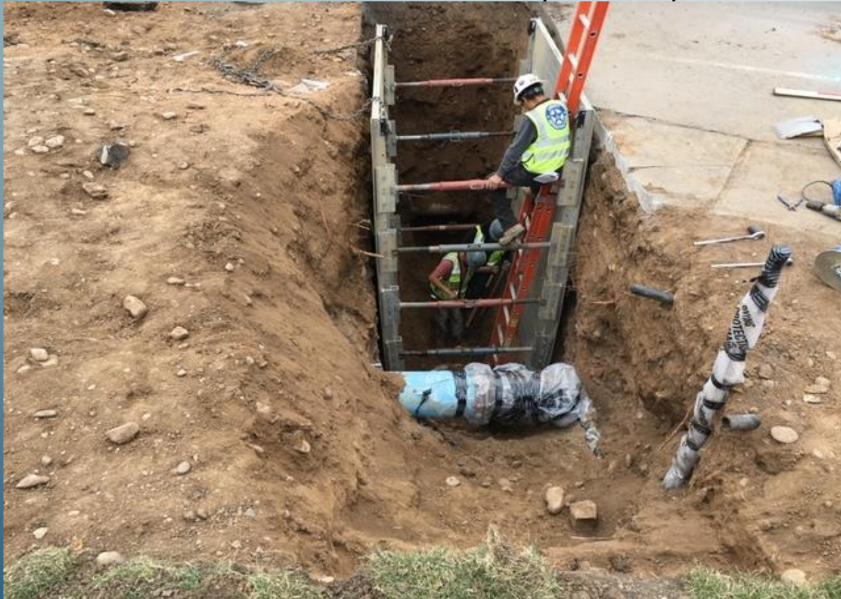
Water main installation in Fairway Lane near SWM connection
