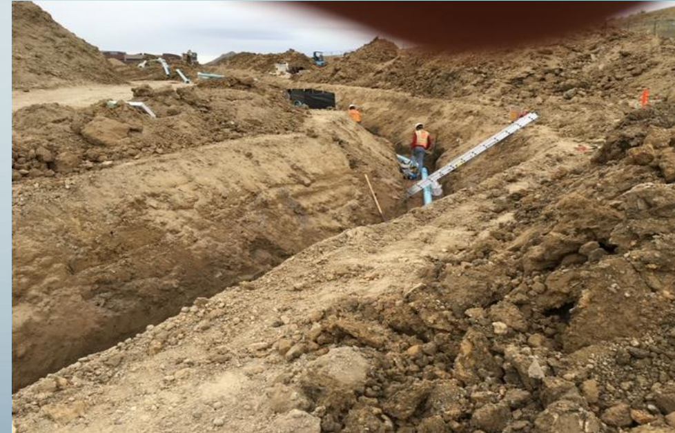
Water Main Trench
