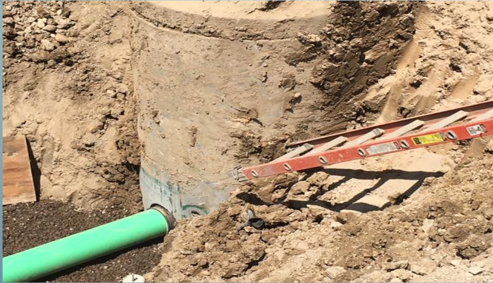
Connection to Existing Manhole
