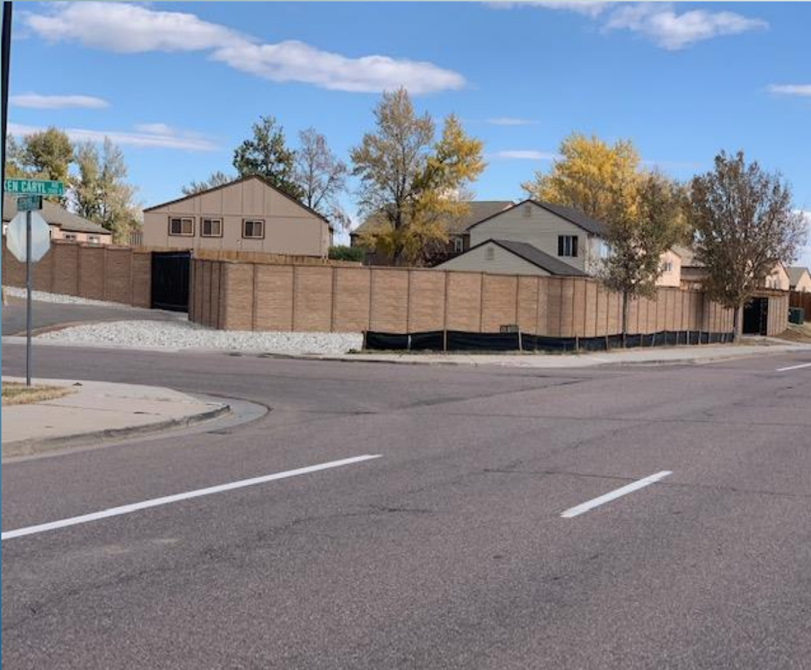
Completed fence and gates
