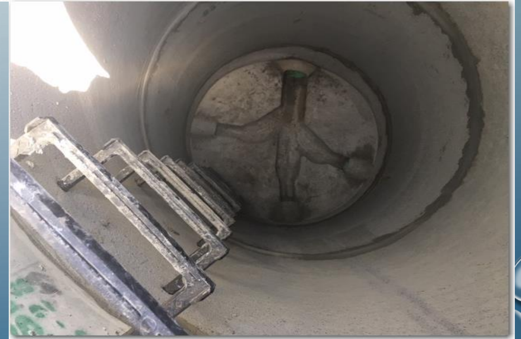
3-Way Service Connection to End Manhole
