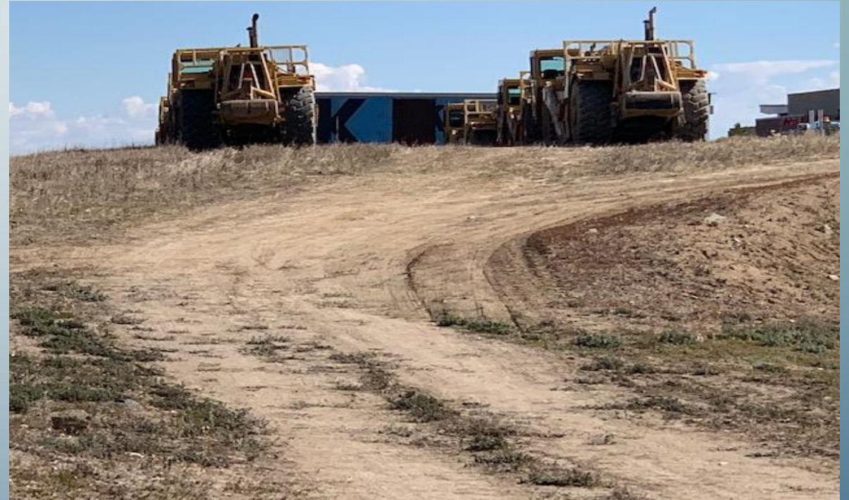
Earth Moving Equipment
