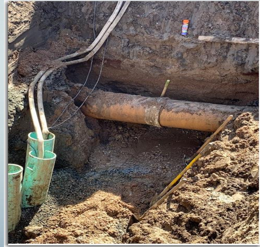
Dewatering; Tie-in at Dutch Ck Interceptor.
