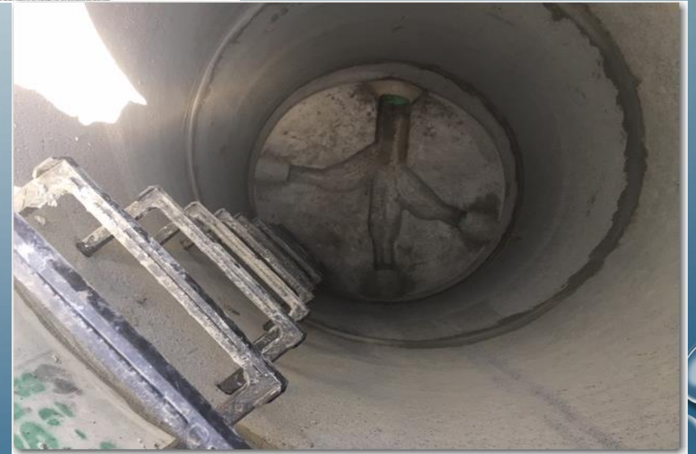
3-Way Service Connection to End Manhole
