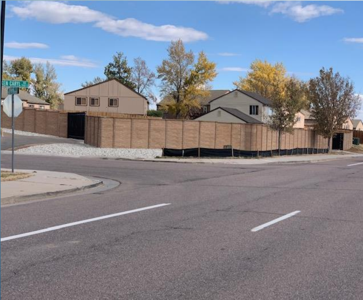
Completed fence and gates
