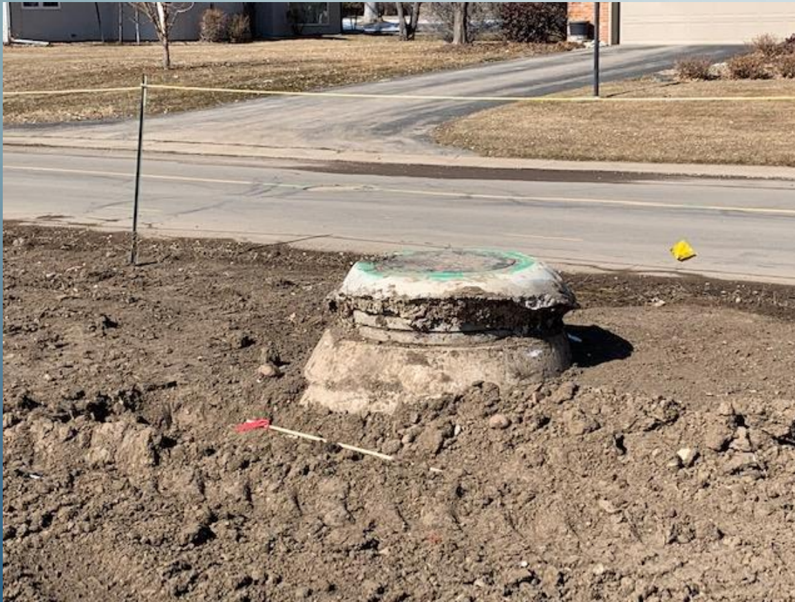
Manholes on B-Line to be lowered
