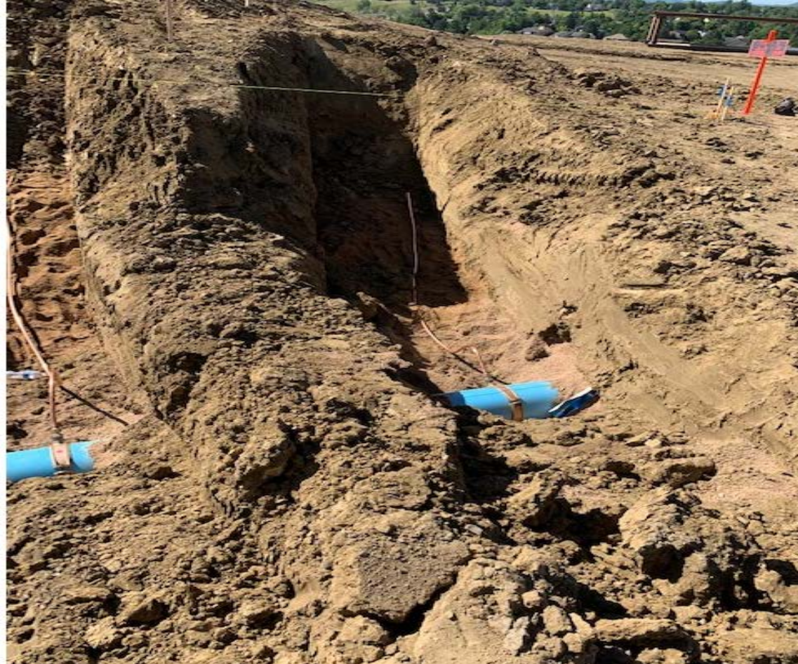
Service lines Stubbed Out of Pavement
