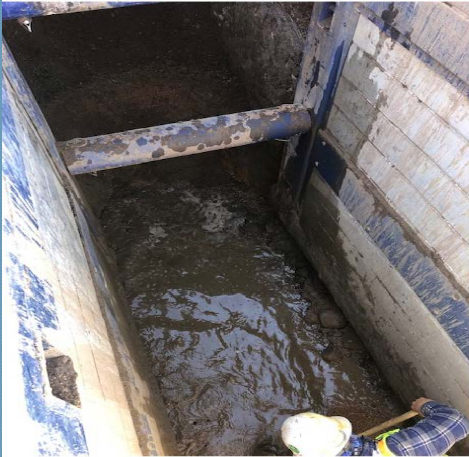
Ground Water in Trench 8' depth
