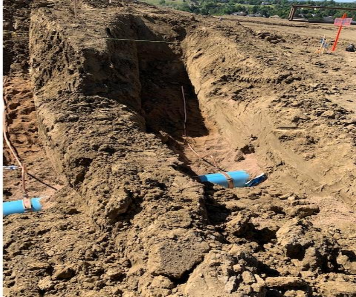
Service lines Stubbed Out of Pavement
