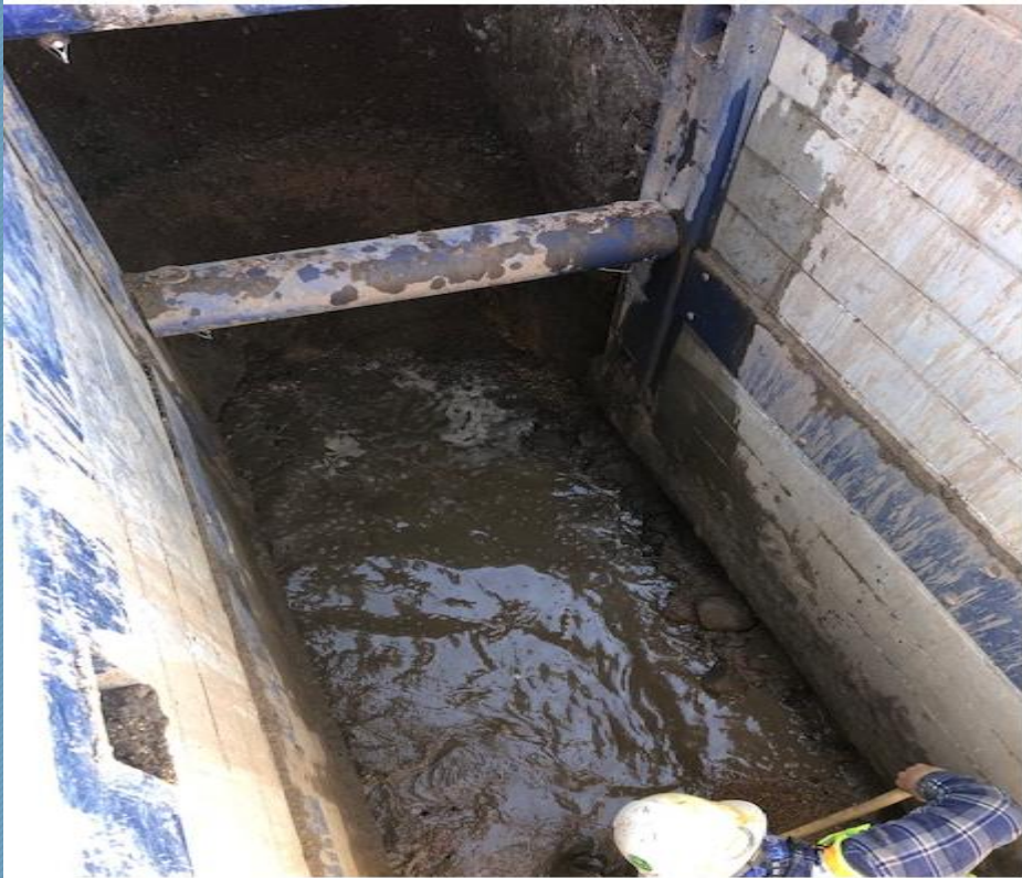
Ground Water in Trench 8' depth
