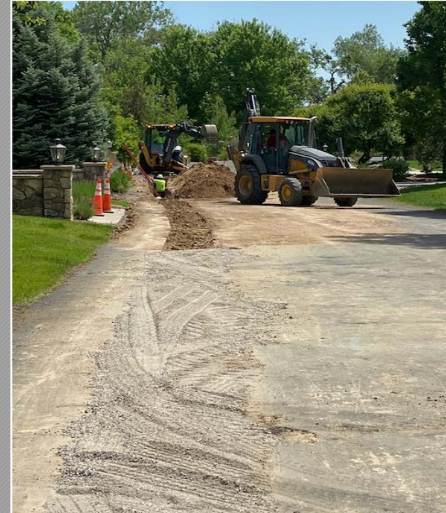
Polo Club 12" Water Trench
