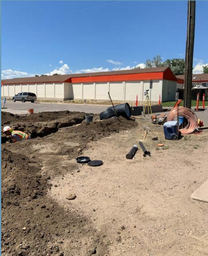
Excavation for the Water Service to Lift Station
