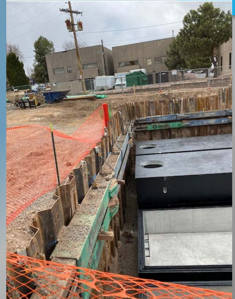
Overflow Tank Installation
