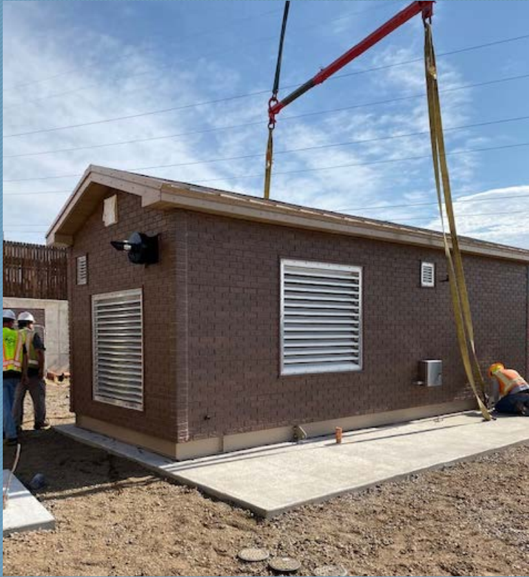
Setting Lift Station on Foundation
