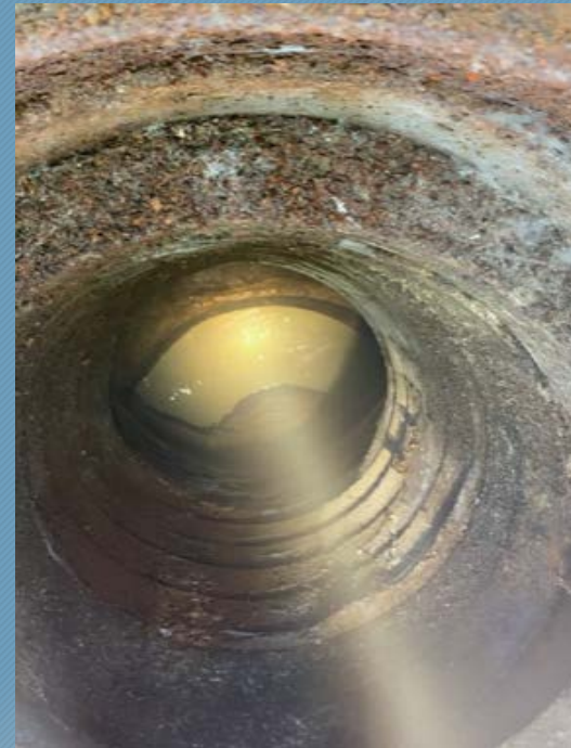
Filled Pipe with Flashfill
