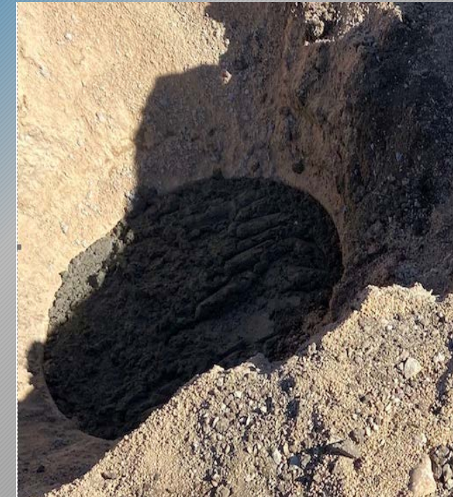
Filled MH W/Squeey and Concrete Cap
