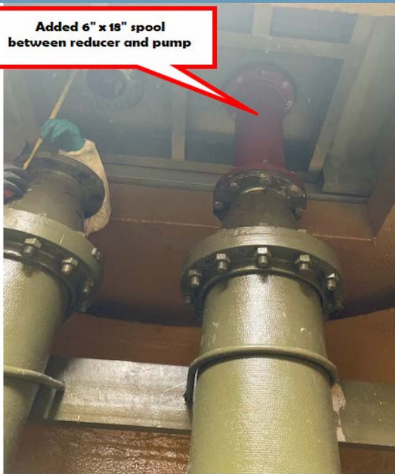
Drained Wet Well - Installed Spool
