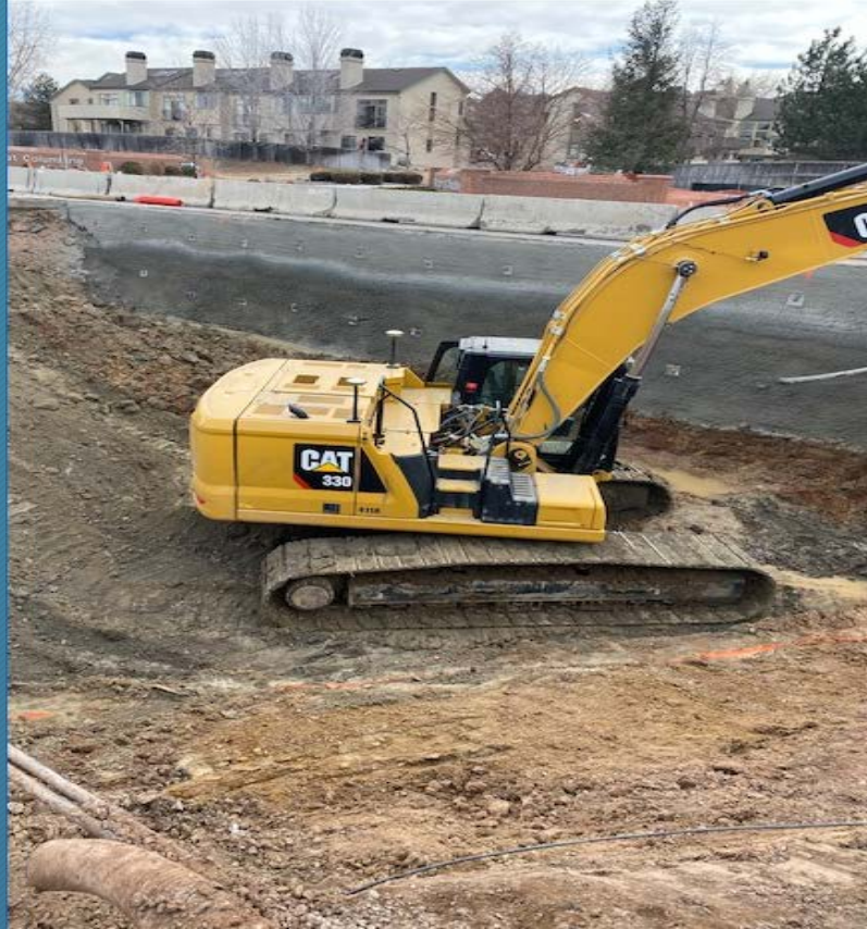
Excavation and Temporary Shoring of Coal Mine Ave East-bound
