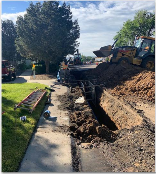
Construction in Depew
