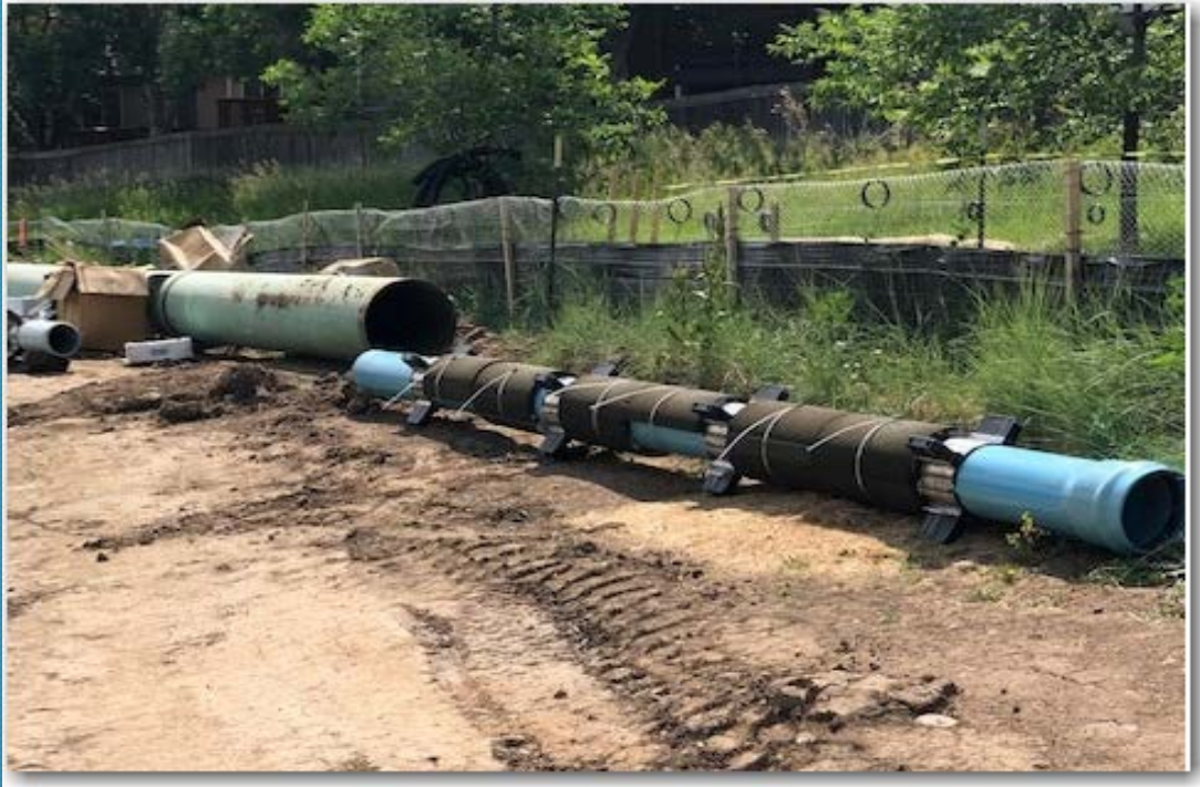
8" Sewer Main with Insulation and Skids
