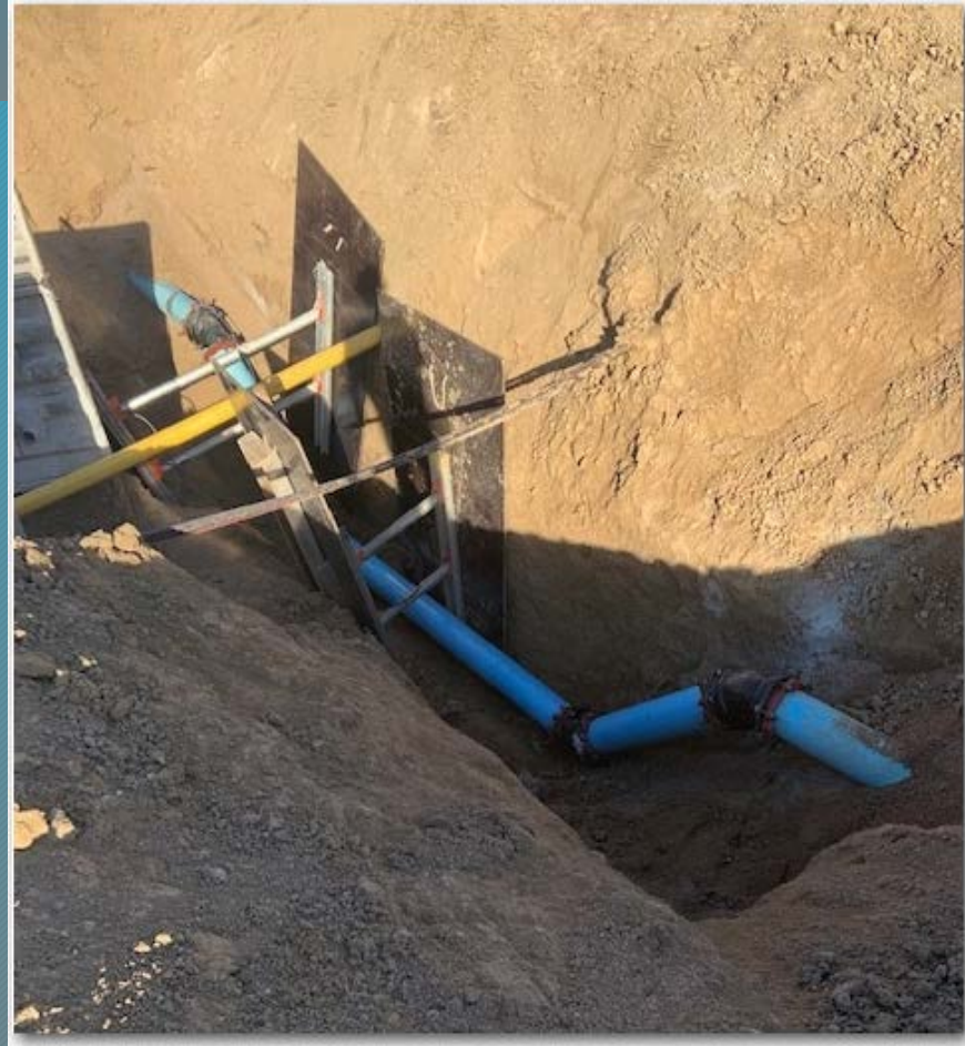
Lowering on New Main for Storm Pipe
