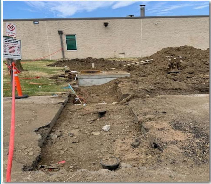
New Domestic Service into Vault
