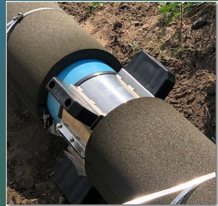
Casing Skid - Supports Pipe in Casing Pipe
