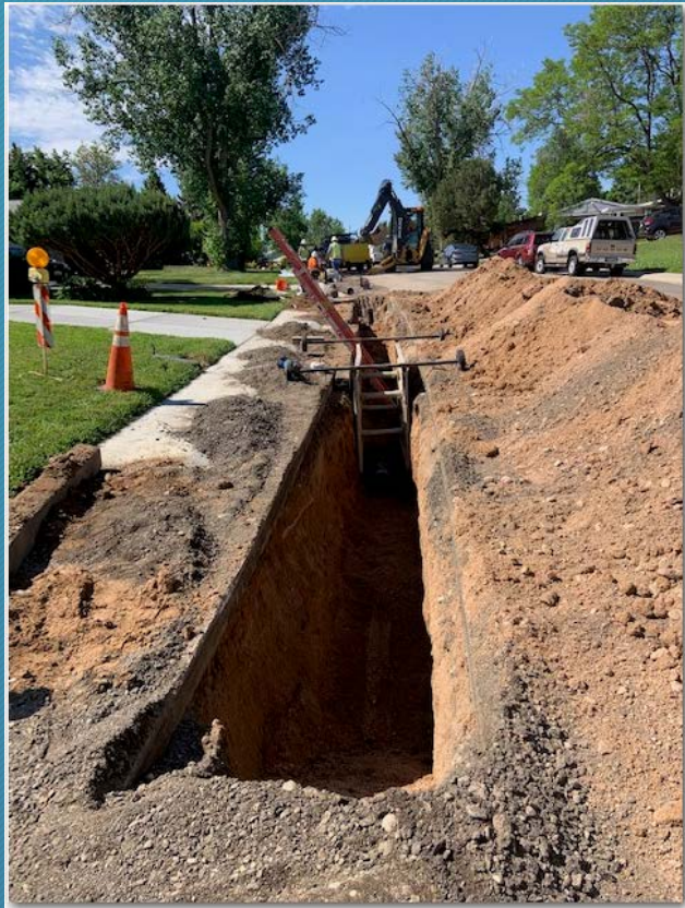
Construction in Depew
