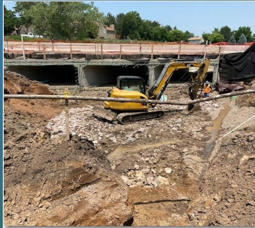
Excavation south side Coal Mine
