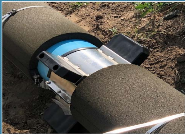
Casing Skid - Supports Pipe in Casing Pipe
