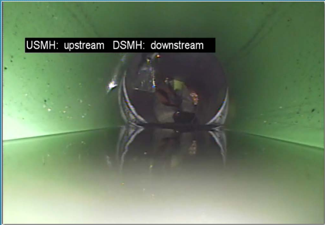
Pre-Video of Dutch Creek Crossing Repair
