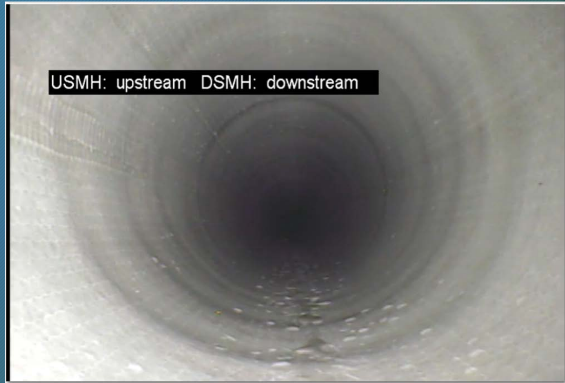
Post Video (New Liner) - Dutch Creek Crossing Repair
