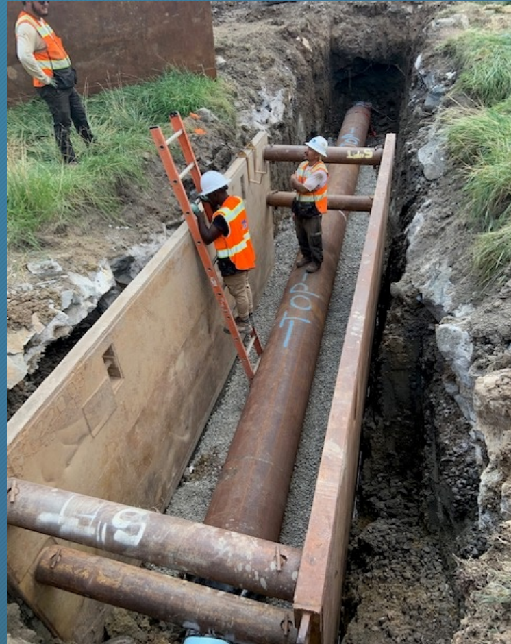
Steel casing in trench
