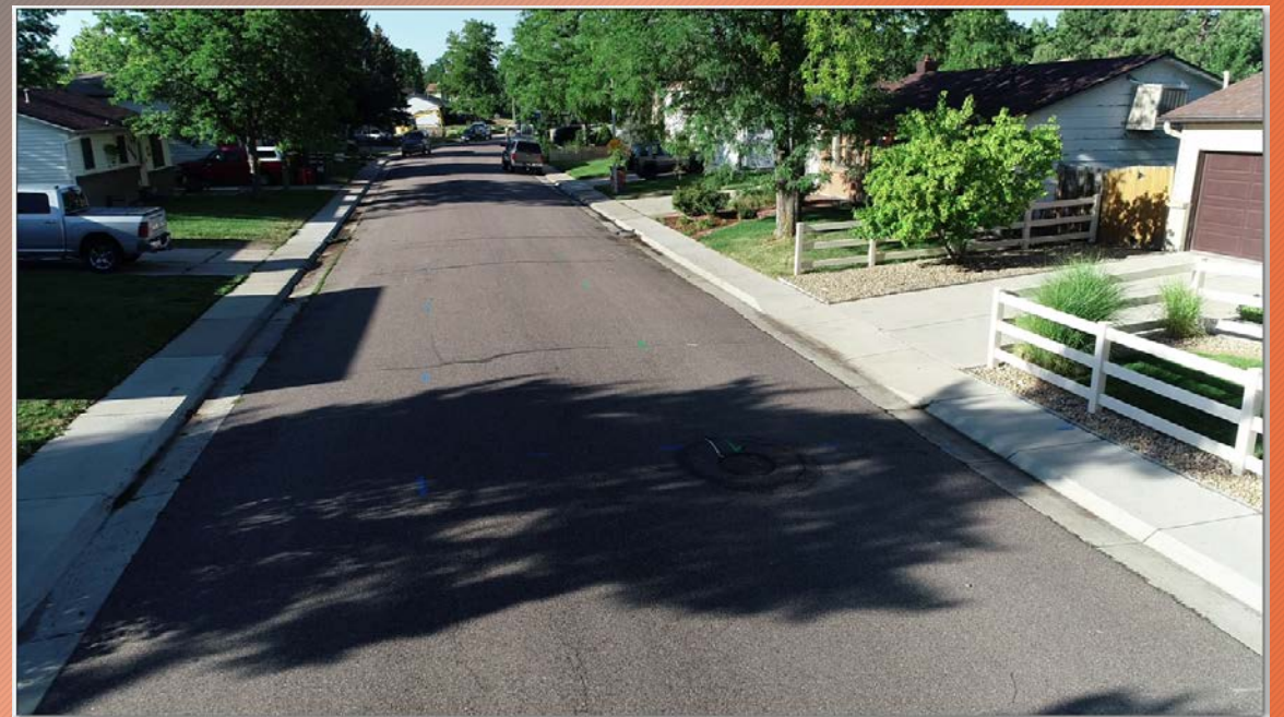
Drone footage of existing conditions i.e. paving and concrete
