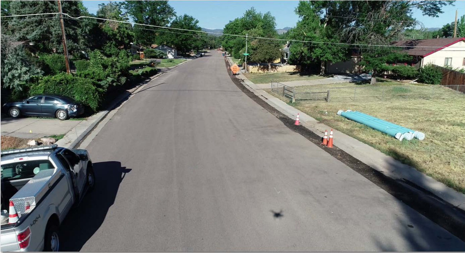
Elmhurst between Lamar and Depew Birdseye view/inspection of trench
