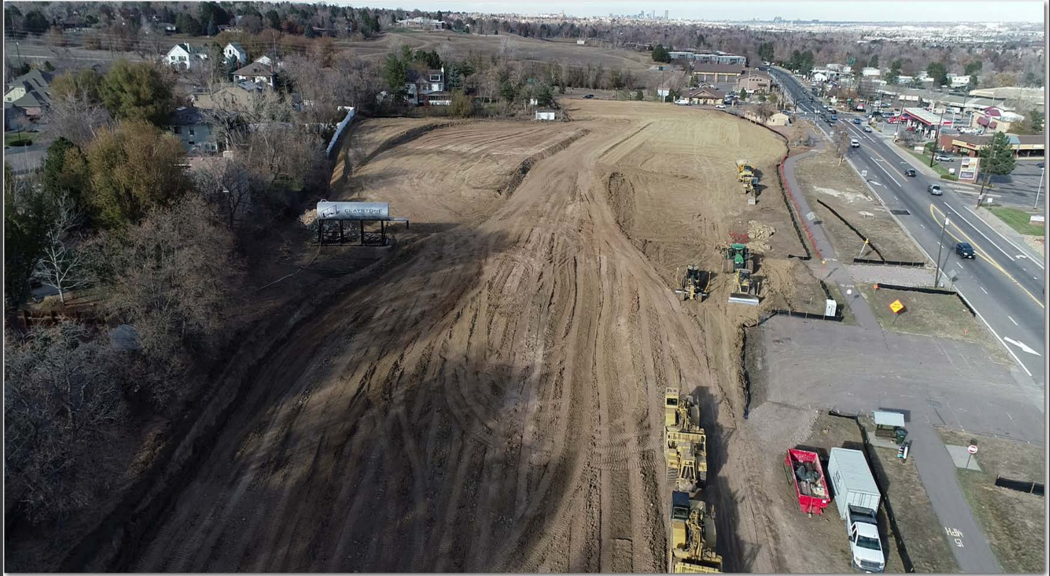
Millstone @ Columbine – After Over-excavation work – site at subgrade
