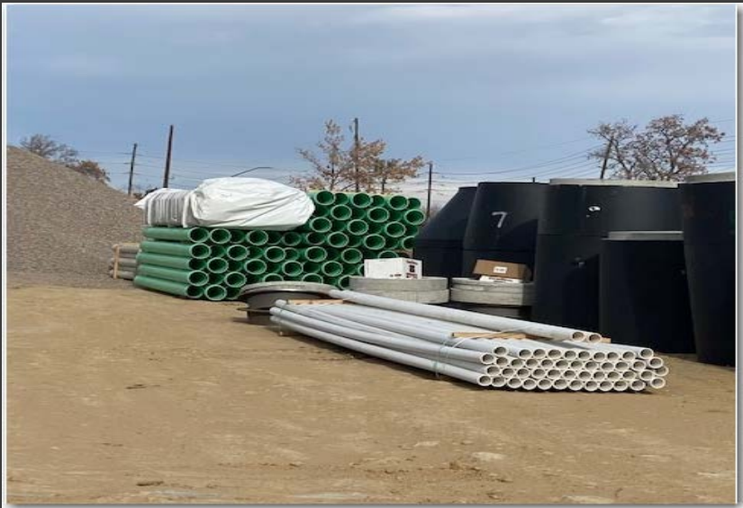
Materials – Sewer Pipe and Manholes on Site
