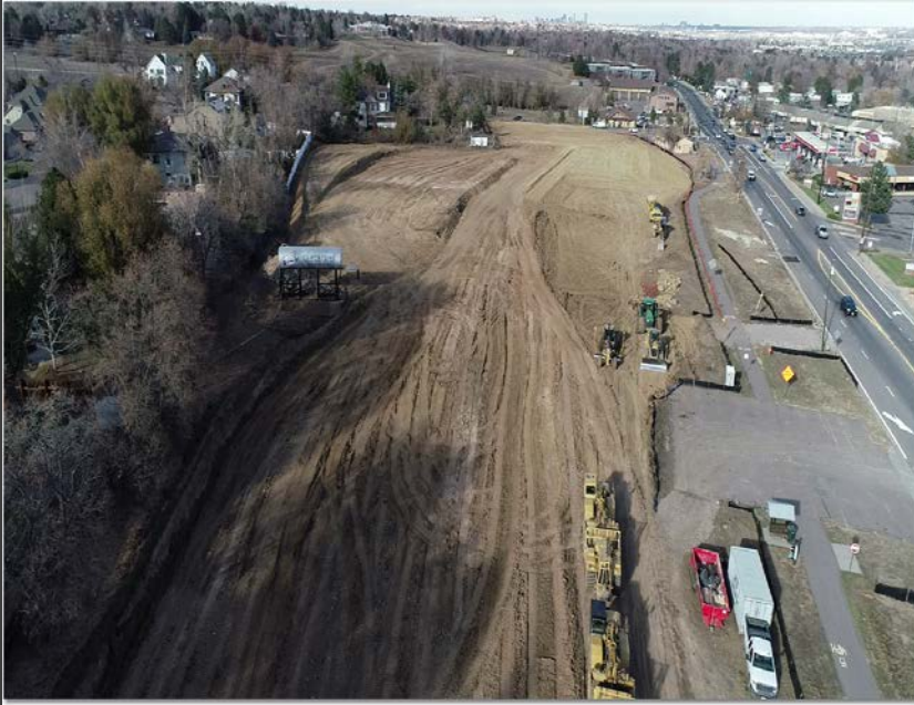
Millstone @ Columbine – over-excavation near completion
