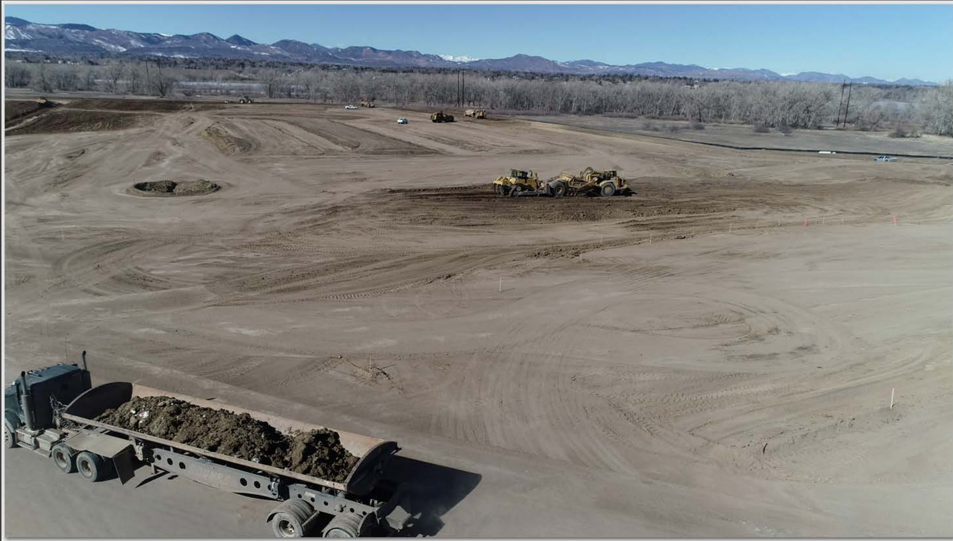
Millstone @ Columbine – Water Main Installation
