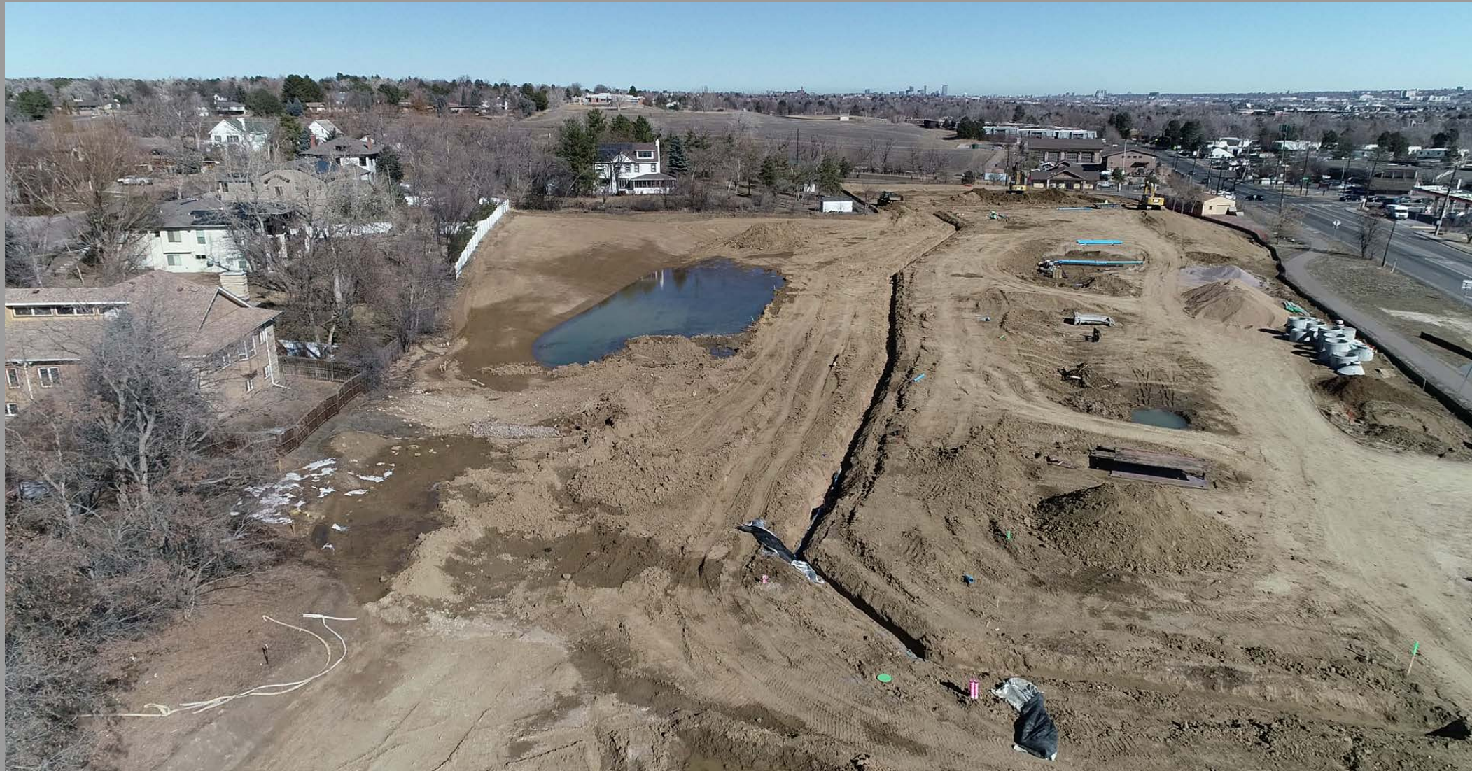
Millstone @ Columbine – Water Main Installation
