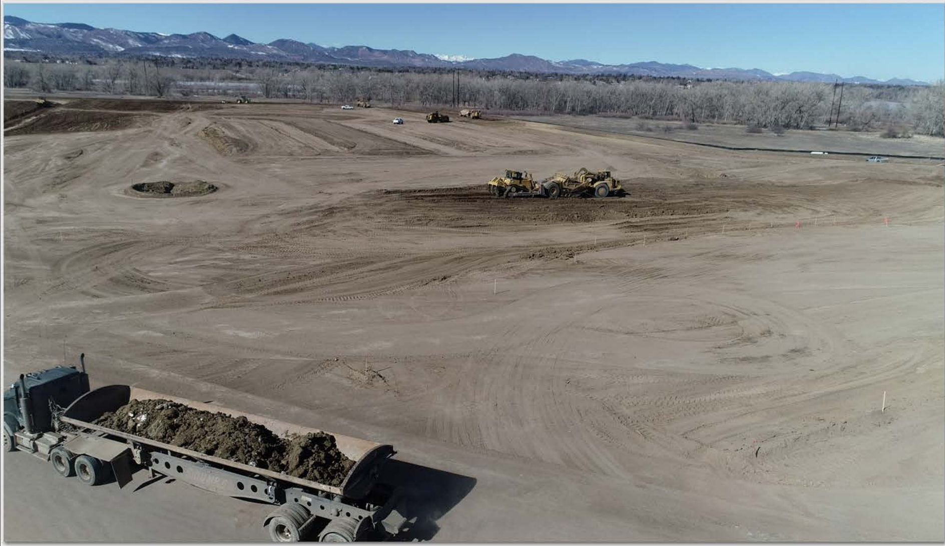
Import Material – D-Line Manhole – To be Raised
