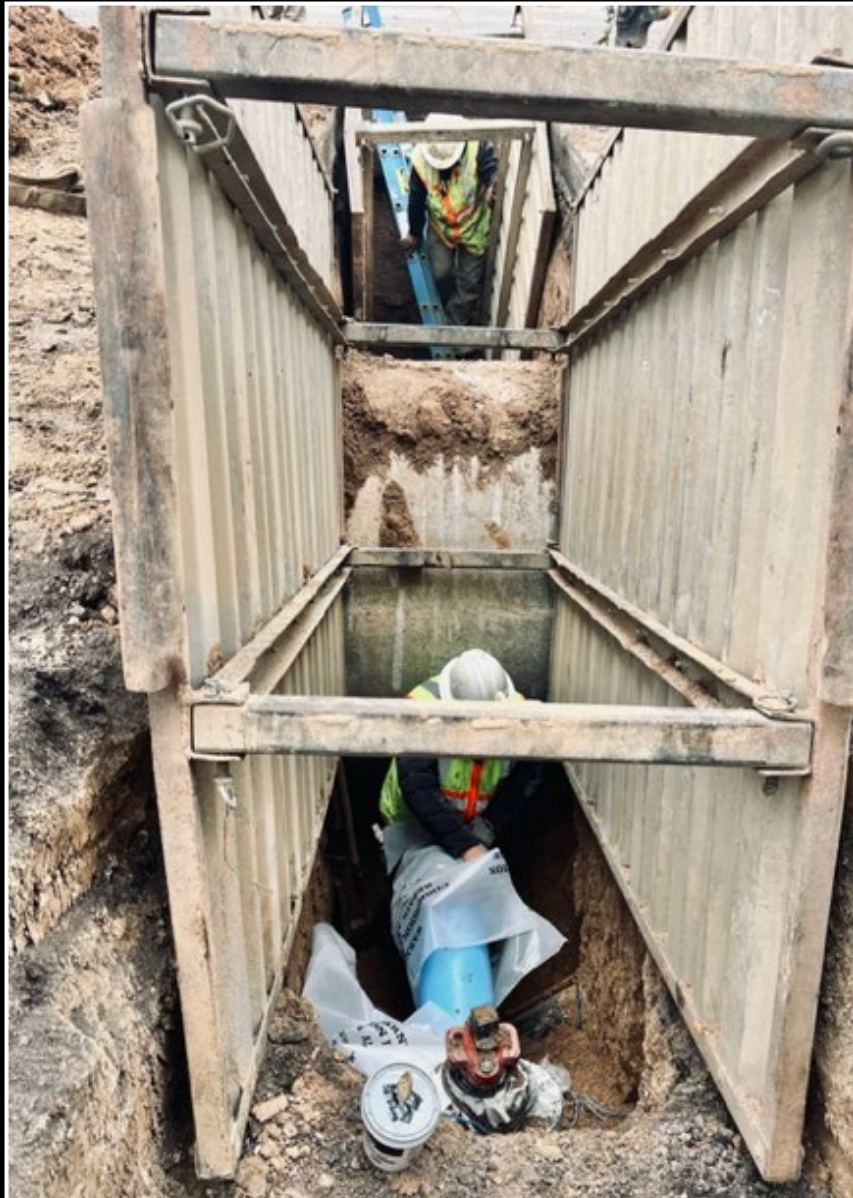
Water main depressed under 60-inch storm on S. Depew St. at W. Caryl Ave.
