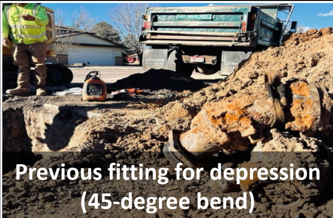
Water main depressed under 60-inch storm on S. Depew St. at W. Caryl Ave.
